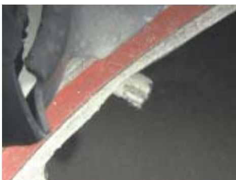
Figure 205: Forward/lower stop pin, overview as viewed from inside.
