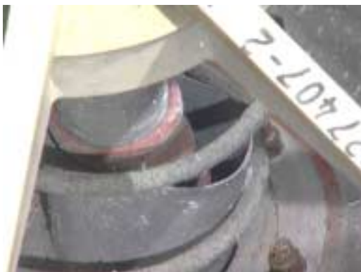
Figure 154: Center diaphragm guide, HS P/N 727411-1, showing distortion of guide itself.
