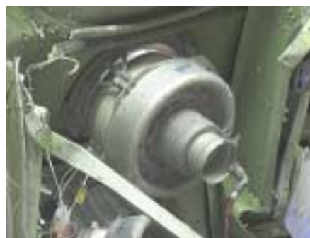
Figure 84: Upper Pressure Relief Valve still installed, as viewed from the inside.
