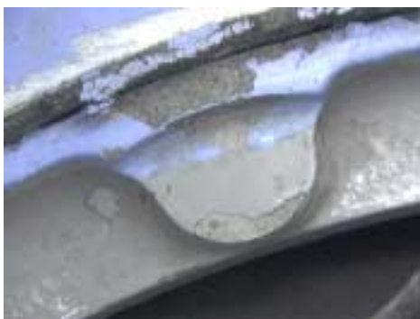
Figure 191 : Upper stop pad; paint chipped.
