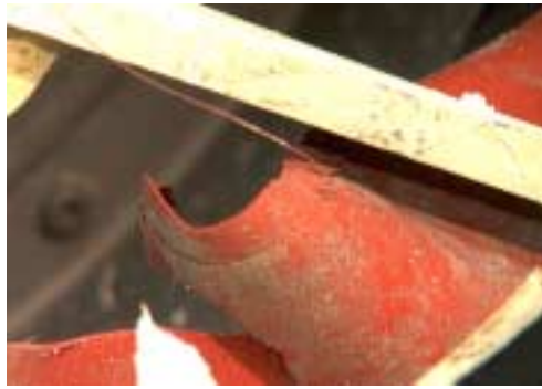
Figure 227 : Outer diaphragm HS P/N 727403-1, torn location.
