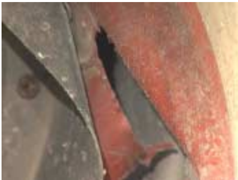
Figure 228 : Outer diaphragm, approximately 60% of circumference is torn.
