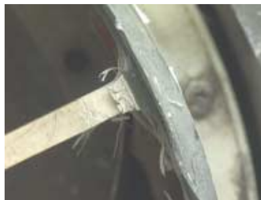
Figure 141: Close-up of knife-edge damage.
