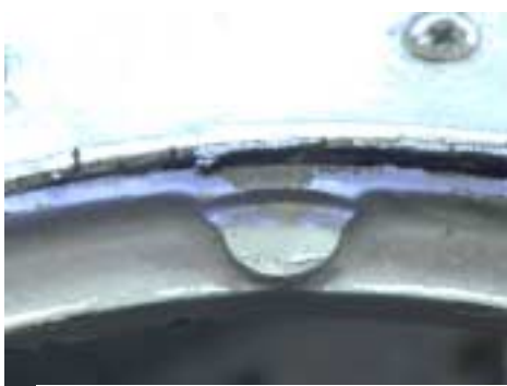
Figure 189 : Exterior opening, close-up, upper door stop pad.
