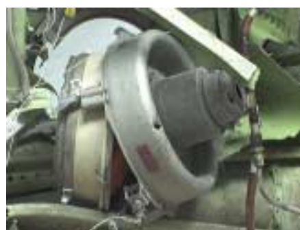
Figure 86: Lower Pressure Relief Valve, still installed, as viewed from the inside.
