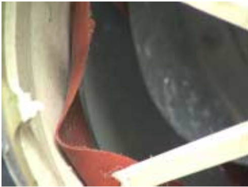
Figure 230: Outer diaphragm damage.
