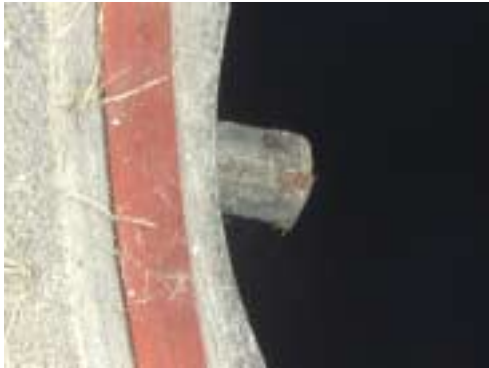
Figure 133: Overview of aft/lower stop pin, as viewed from inside.
