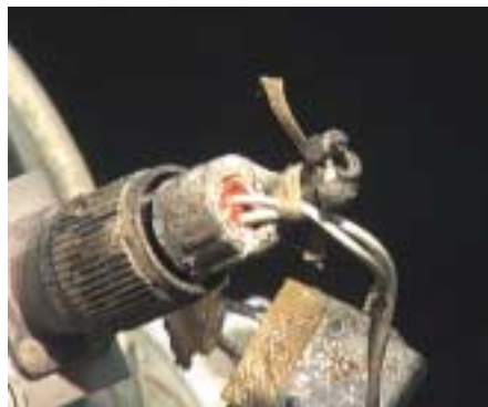
Figure 210: Electrical switch connector interface appears to be intact.
