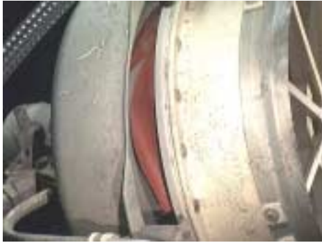
Figure 148: Diaphragm, circumferential tear.
