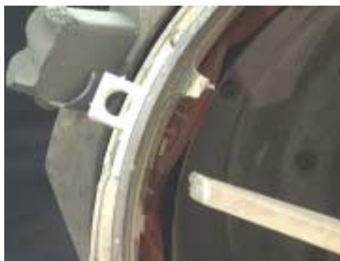
Figure 217: Broken web detail.
