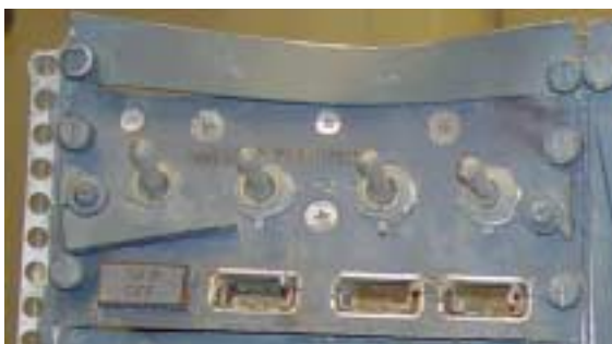
Figure 52: Galley Power control panel M179 • Light plate is missing. • All switch toggles are in up position. • TRIP OFF indicator lights, numbers 2, 3 & 4 legend plates, bulbs and retaining assemblies are missing.
