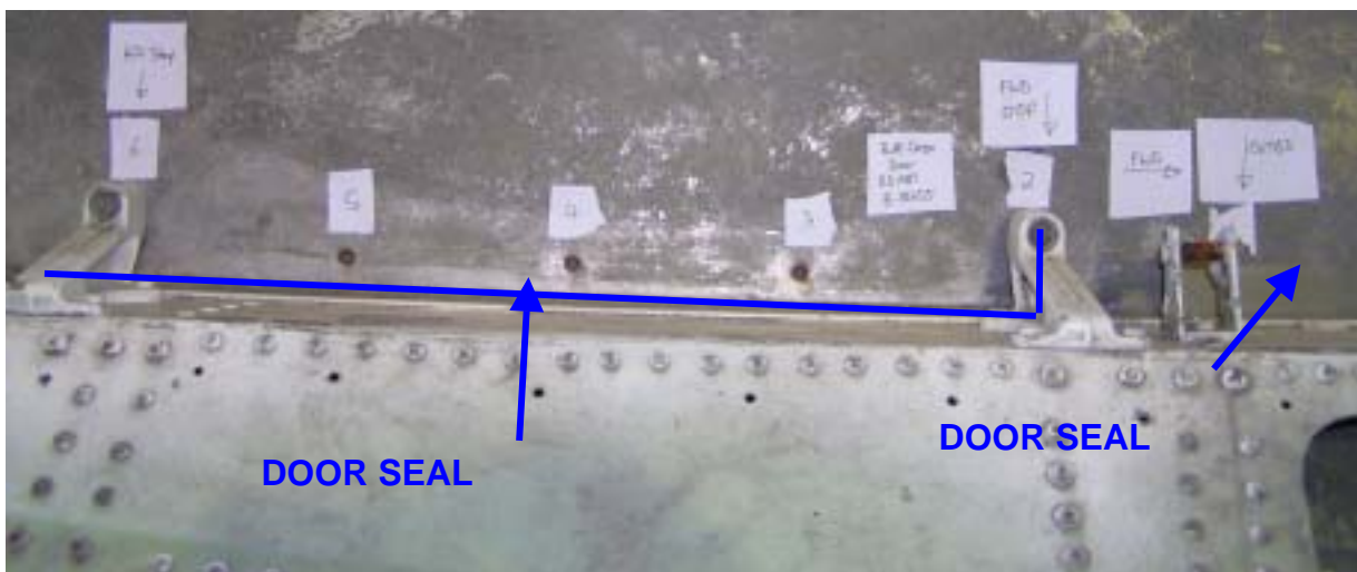
Figure 1.12-80 Interior View of Lower Edge of Bulk Cargo Door
