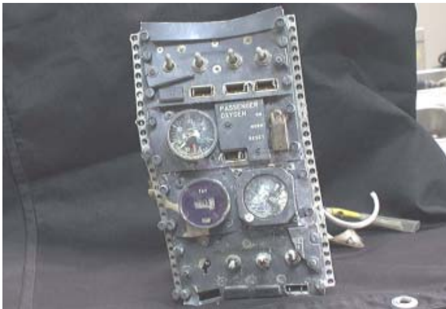
Figure 1.16-4 Partial Flight Engineer's Panel
