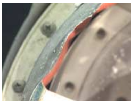
Figure 139: Close-up of knife-edge damage.
