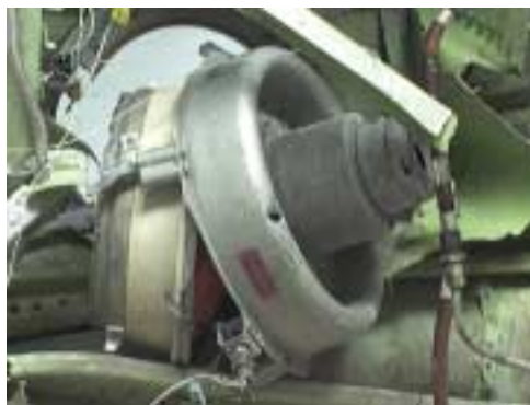
Figure 177: Lower Pressure Relief Valve as viewed from inside, still installed but not attached to structure. (Ref. For following section on pins and stops)
