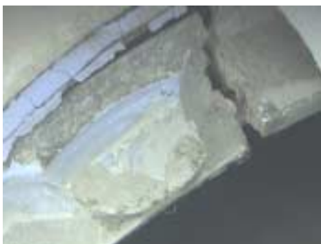
Figure 200: Lower stop pad, with adjacent crack on housing.
