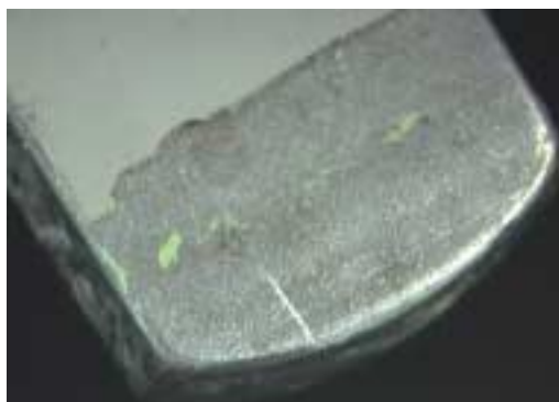
Figure 199: Forward/upper stop pin, close-up of figure #198. • Paint is chipped.
