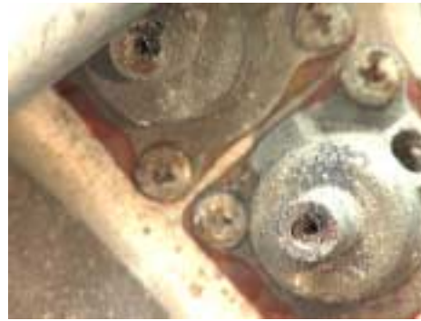
Figure 242: Control adjustment screws, both appear to be intact.
