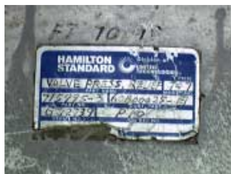
Figure 175: Lower Pressure Relief Valve, data plate identification.
