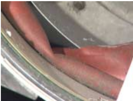
Figure 146: Diaphragm, showing typical tear.
