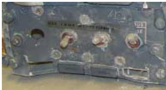
Figure 67: DC BUS ISOLATION panel, module M557
