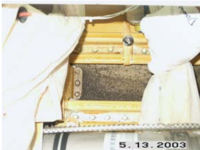
Figure 1.6-7 A bilge without removing the corrosion preventative compound
