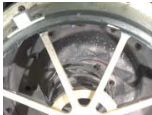
Figure 155: Gate return spring, showing unseated spring.
