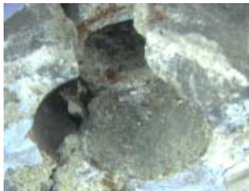
Figure 187 : Forward/upper hinge pin, close-up of partial bushing.
