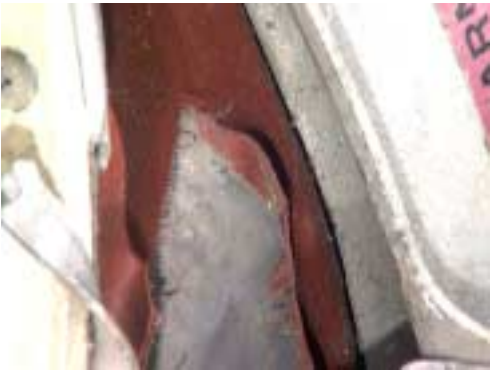
Figure 233: Outer diaphragm, close-up of tear origin.
