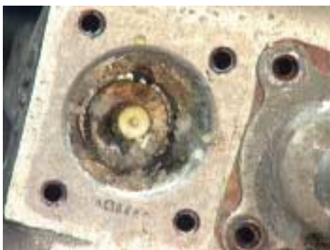
Figure 251: Close-up of salt deposits inside housing bore.
