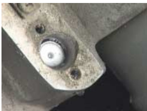
Figure 169: Shows water in plug area.
