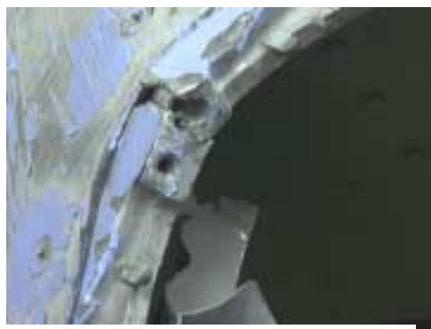
Figure 185 : Exterior opening, close-up, another view of figure #184
