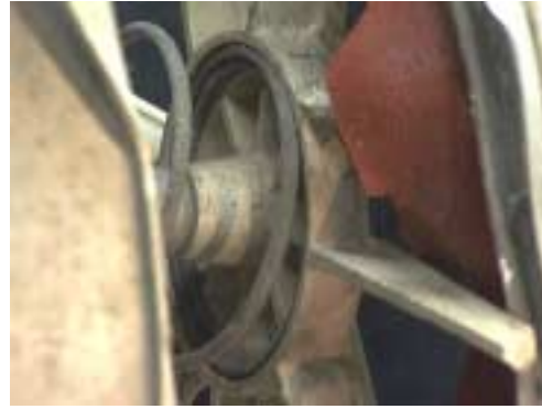
Figure 237: Gate return spring is seated in the gate. The end coil appears to be inside the last active coil.
