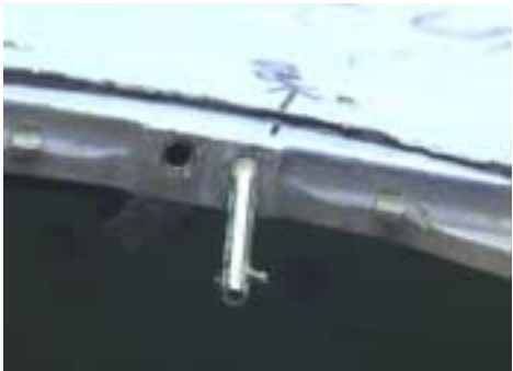
Figure 104: Forward/upper hinge pin, physically rotated by hand to bend inboard.
