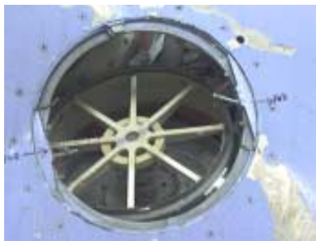
Figure 82: Upper Pressure Relief Valve, close-up showing markings.
