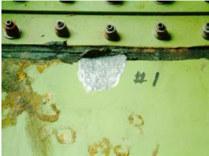
Figure 1.16-139 Higher magnification of #1 corrosion pit, after cleaning (0.99X)
