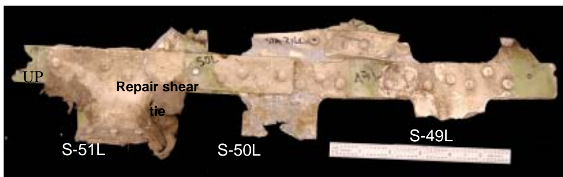
Figure 1.16-106 As received condition of the STA 2160 frame segment submitted for examination. The forward surface is shown in this view.
