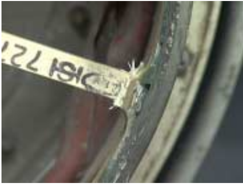
Figure 142: Overview, close-up of typical web fracture.
