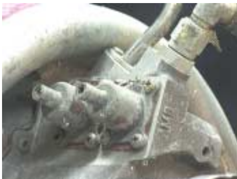
Figure 240: Control assembly area (sense housing area), overview. • Intact, some surface accumulation. • Nothing looks out of place. • Integral ambient sensing tube attachment looks normal. • Remote tube attachment looks normal.
