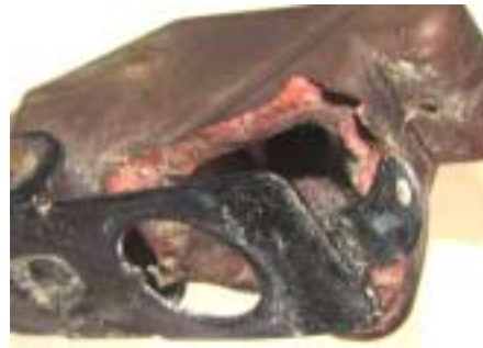
Figure 62 : Bottom view of switch guard damage.
