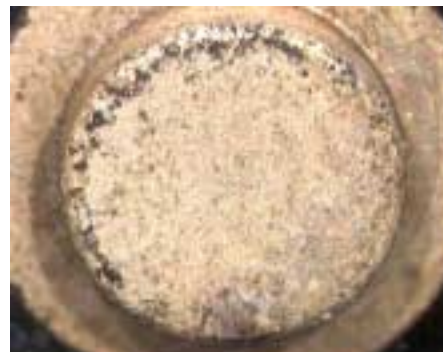
Figure 58 : Stationary contact of oxygen control switch ("RESET" position).
