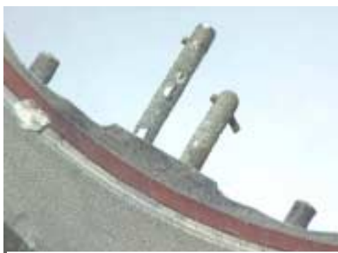
Figure 108: Close-up of aft stop & hinge pins (looking from inside out).
