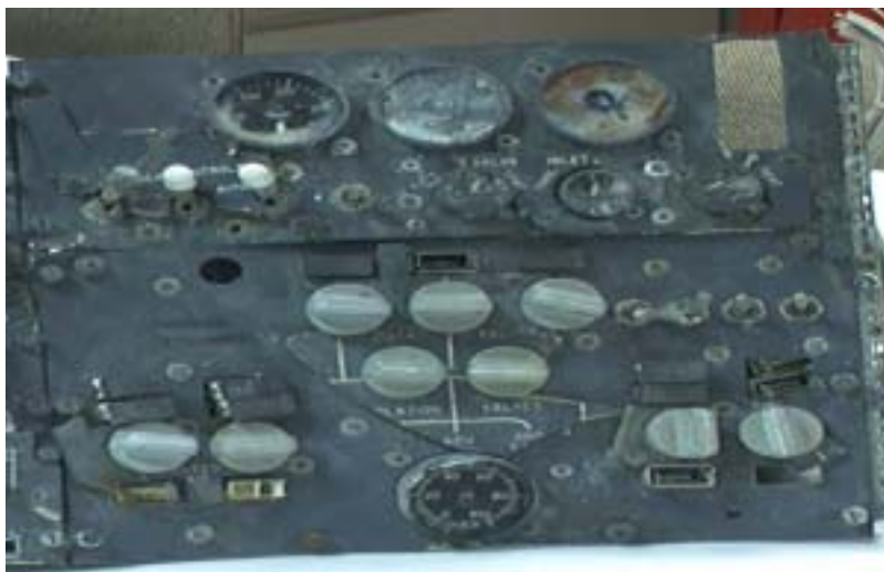
Figure 1.16-2 Air Conditioning Panel
