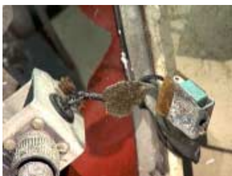
Figure 213: Switch lead wires showing bond detached from housing.
