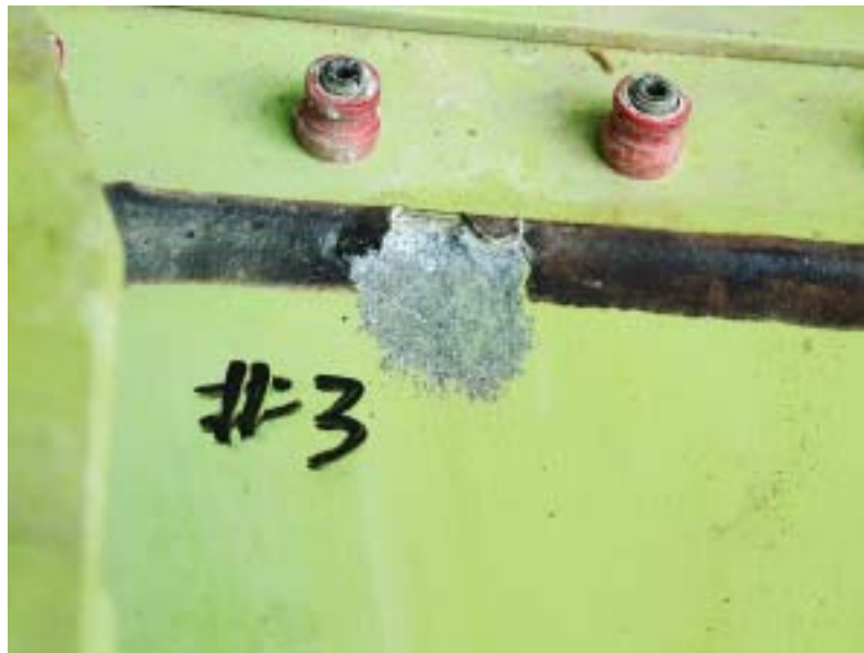
Figure 1.16-141 Higher magnification of #3 corrosion pit, after cleaning (1.73X)
