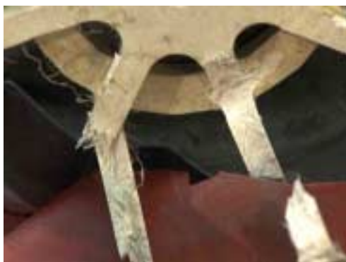
Figure 216: Gate webs, detailed view of broken web members.
