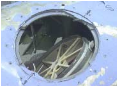
Figure 90: Exterior view of opening with valve not yet removed.
