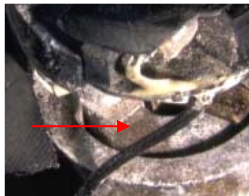
Figure 20: RIGHT, OUTFLOW VALVES Indicator; armature moved to show witness mark.
