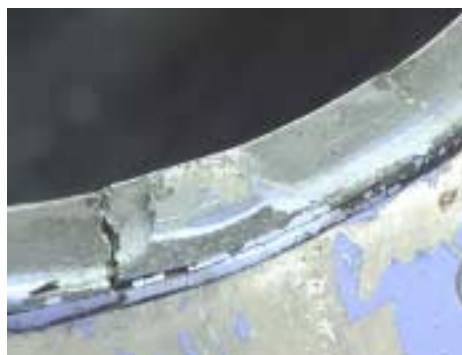
Figure 190 : Exterior opening, close-up, upper door stop pad.
