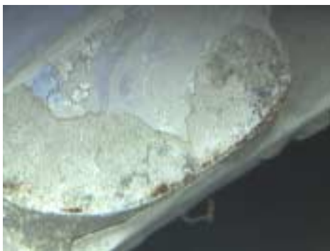
Figure 202: Close-up of figure #200, paint chipped.
