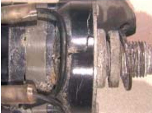
Figure 30: Switch #3 body crack detail • Corrosion on all metallic parts • Severe cracking of the switch body. • No continuity could be attained. • All external wiring appears intact. • X-ray shows that the valve-closed electrical contacts are not aligned with each other. Misalignment approximately 10 degrees. The switch knob was not in the full closed position.
