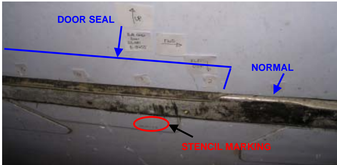
Figure 1.12-81 Exterior View of Bulk Cargo Door Lower Edge
