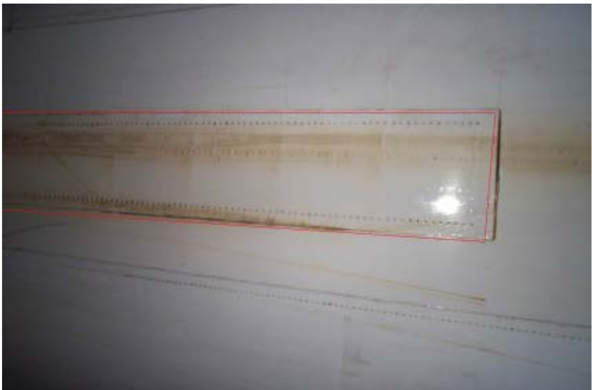
Figure 1.6-5 Number 16 doubler and surroundings ( Picture taken at 6C on Nov 26,2001
