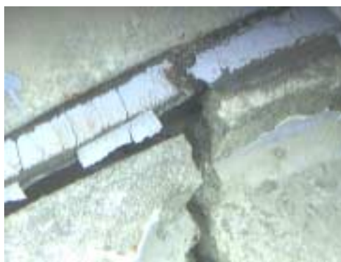
Figure 201: Detail of lower stop pad. • It is broken away from housing (housing cracked).
