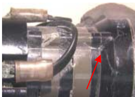
Figure 34: Bleed Air Switch #1.
