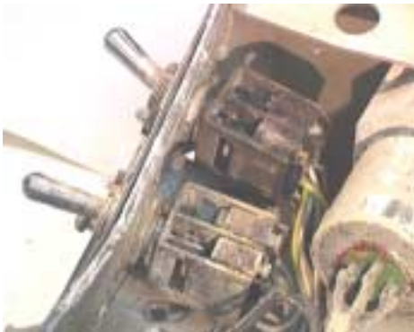
Figure 22: Outflow Valves, MANUAL CONTROL, OPEN & CLOSE toggle switches as viewed from underneath.
