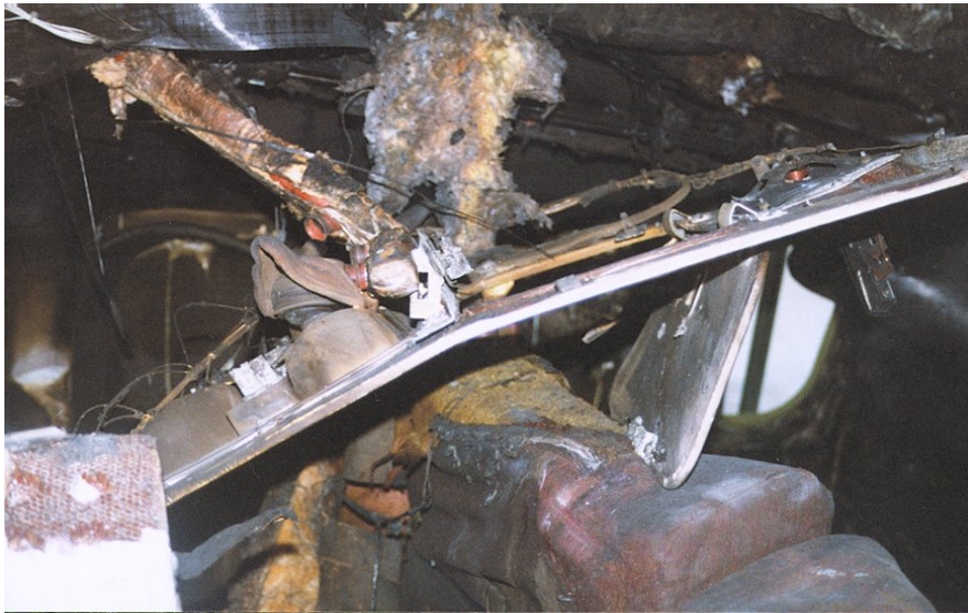
Fig. 1.12-13 Condition of the PSU
