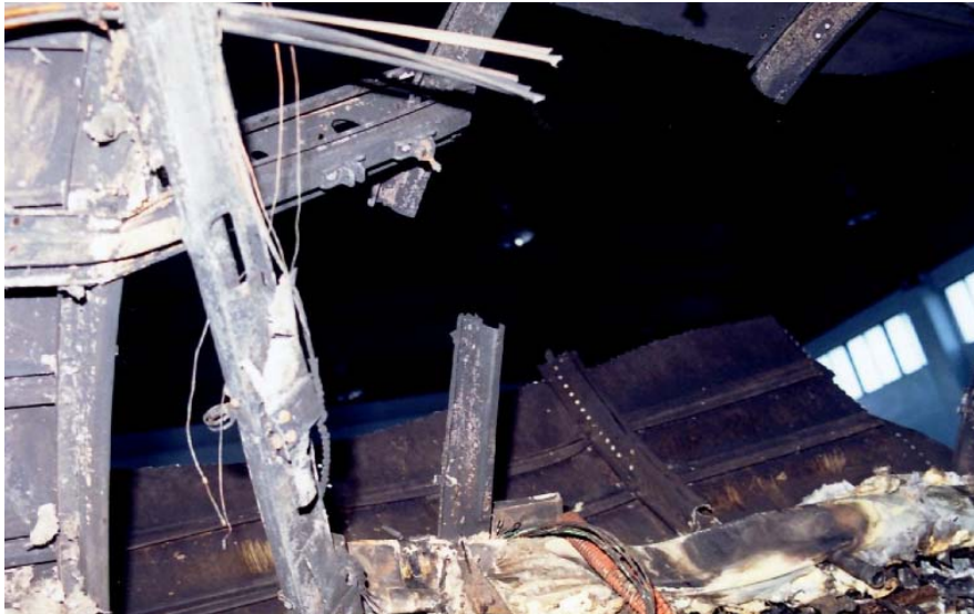
Fig. 1.12-8 Breaking point of the longitudinal beam
