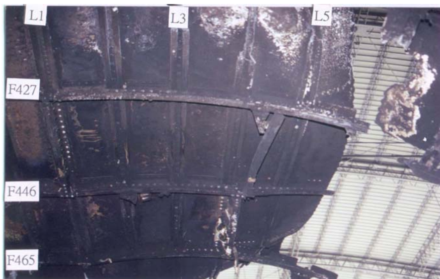
Fig. 1.12-5 Ripped-off structural skin in the vicinity of the framework
