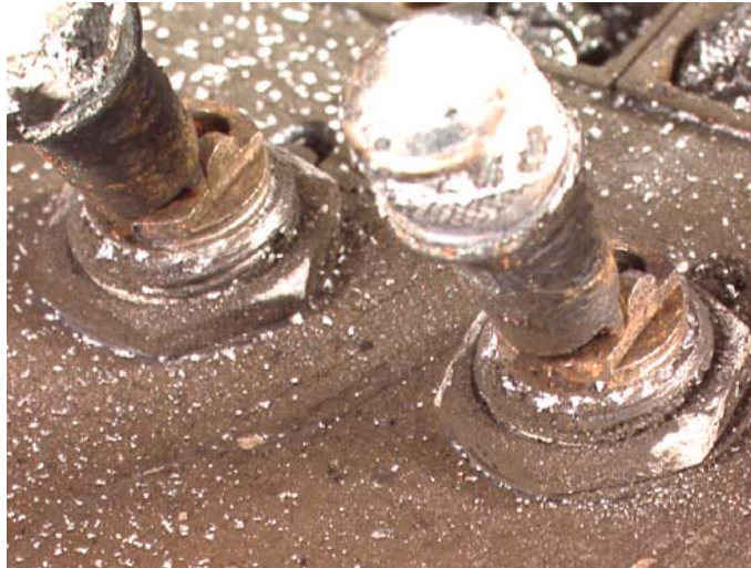
Figure 6. The Position of Toggle Switches Located on the Right of the Fuel Control Panel
