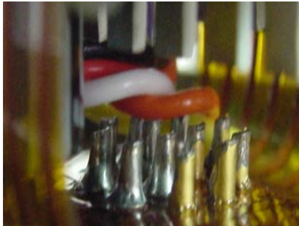
Figure 16. Wires Resting on Sharp Solder Cups in Right Gauge
