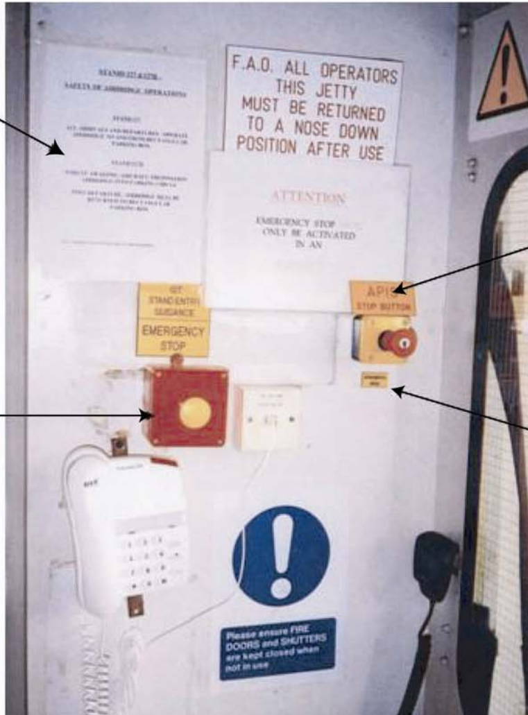
View illustrating confusing nature of displayed information/emergency stop buttons on Stand 127
