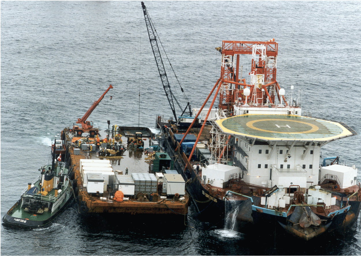
Figure 18: Heavy lift operation
